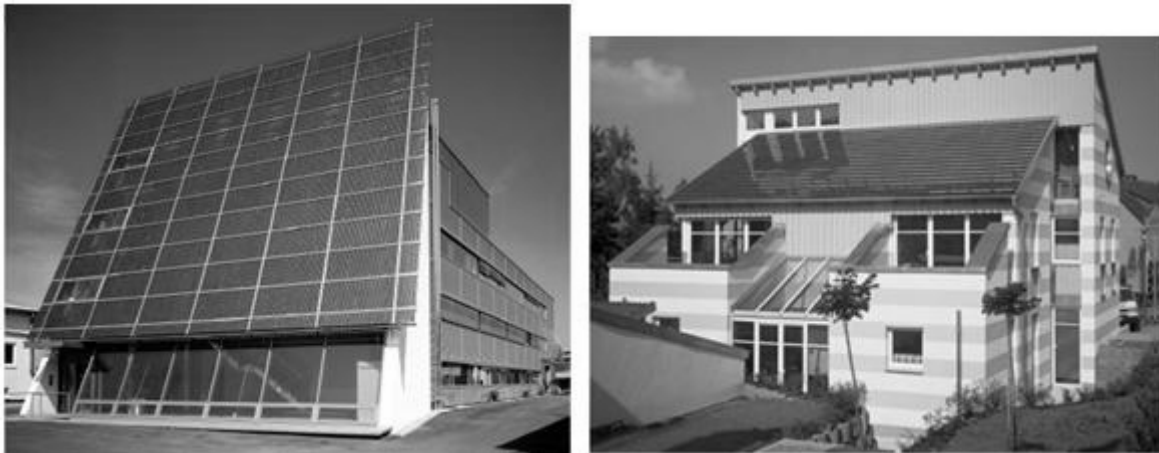
Figure 1-1: BIPV Examples, buildings in Germany
