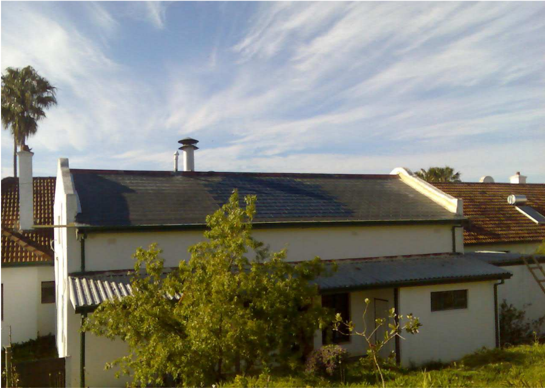
Figure 7-2: Shadow of chimney on PV panels
