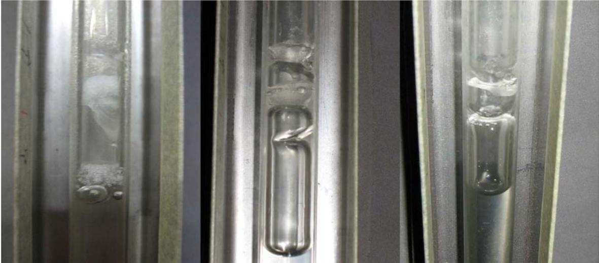
Figure 5.11: Ice in the evaporator sight glass
