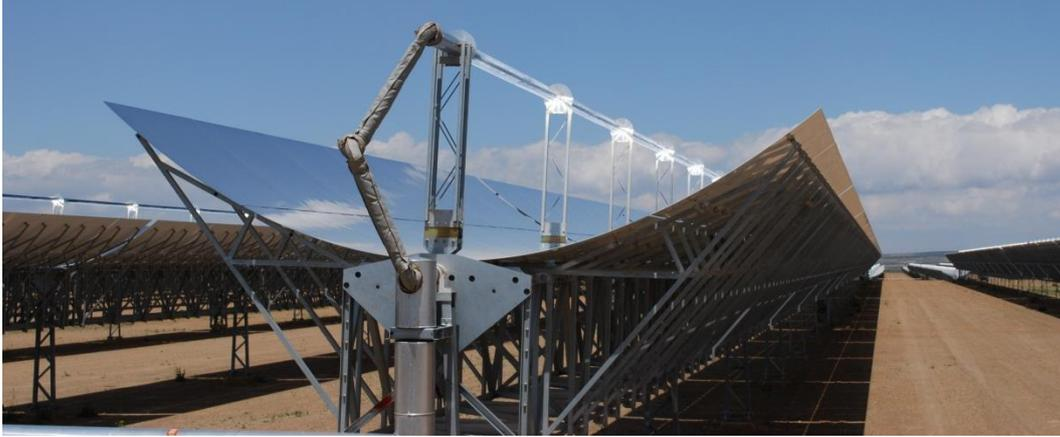
**Figure 2.8: Photo of a parabolic trough line in Andasol 3, a 50 MW parabolic trough plant with 7.5 hours of storage (Photo by author)**
