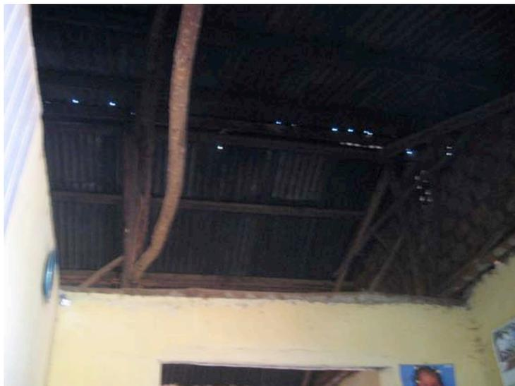
**Figure 111: None of the houses had ceilings installed. By installing ceilings, more light could be refracted and used within the desired area.**
