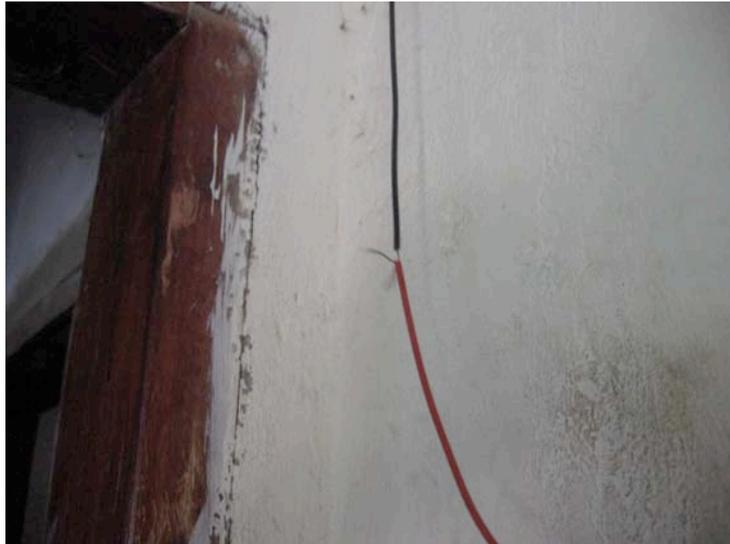
**Figure 112: A contact to switch on and of the white LEDs in a room. Such weaknesses in the system installation reduced the sustainability of the project.**
