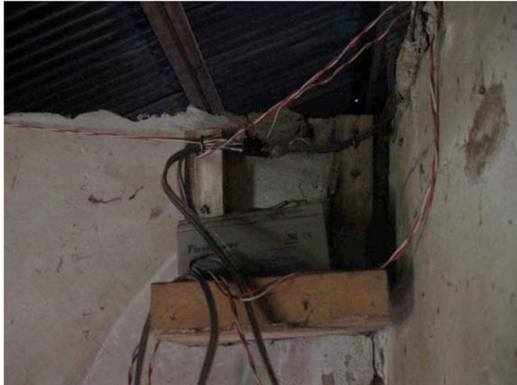
**Figure 110: The battery used to store charge from a solar PV system**
