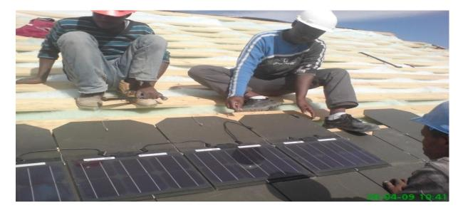
Figure 4.3: Builders installing solar PV roof tiles at Lynedoch Eco-village
