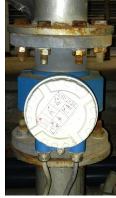
(b) Electromagnetic flow meter
