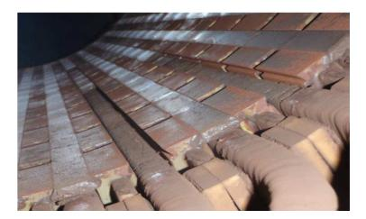
Figure 27: Missing stator slot wedges
