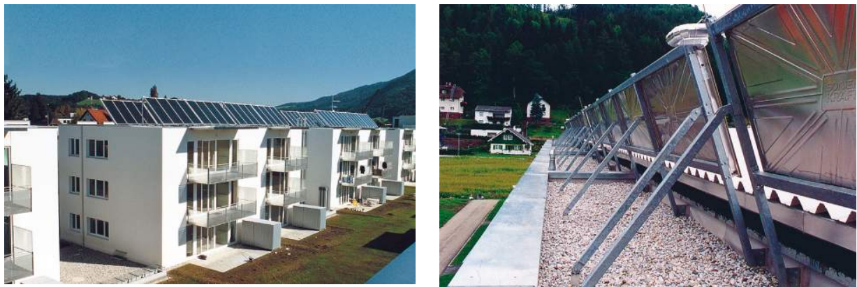
Figure 56: Collectors mounted on a flat roof (Source: Solution Solartechnik), (9,10)
