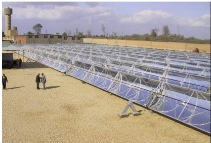
Figure 111: El NASR Pharmaceutical Chemicals, Egypt. Installed capacity: 1,33 MW th Source: Fichtner Solar GmbH. Germany.
