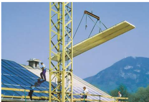
Figure 53: (left) Crane assembly of large-area collectors (picture source: S.O.L.I.D., Austria). Figure 54: (right) Crane assembly of the entire roof elements with support construction and collector field (picture source: Wagner & Co, Germany).
