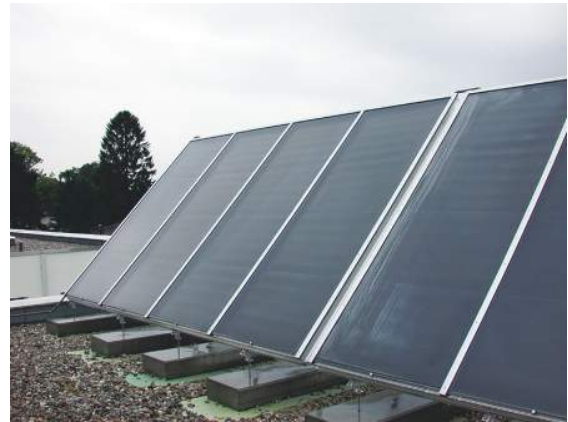
Figure 57: Collectors mounted with different mounting techniques on flat roofs
