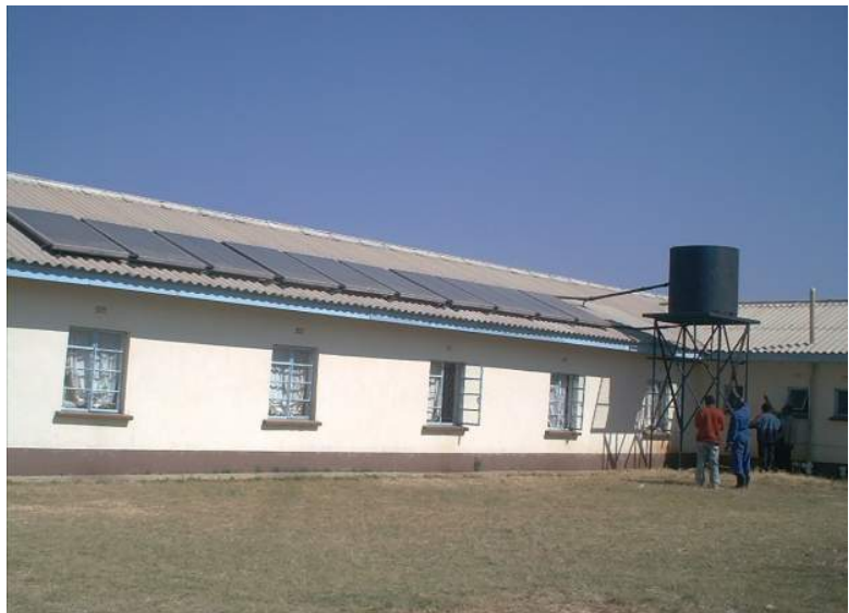
Figure 86: Simple direct thermosyphon systems, Zimbabwe
