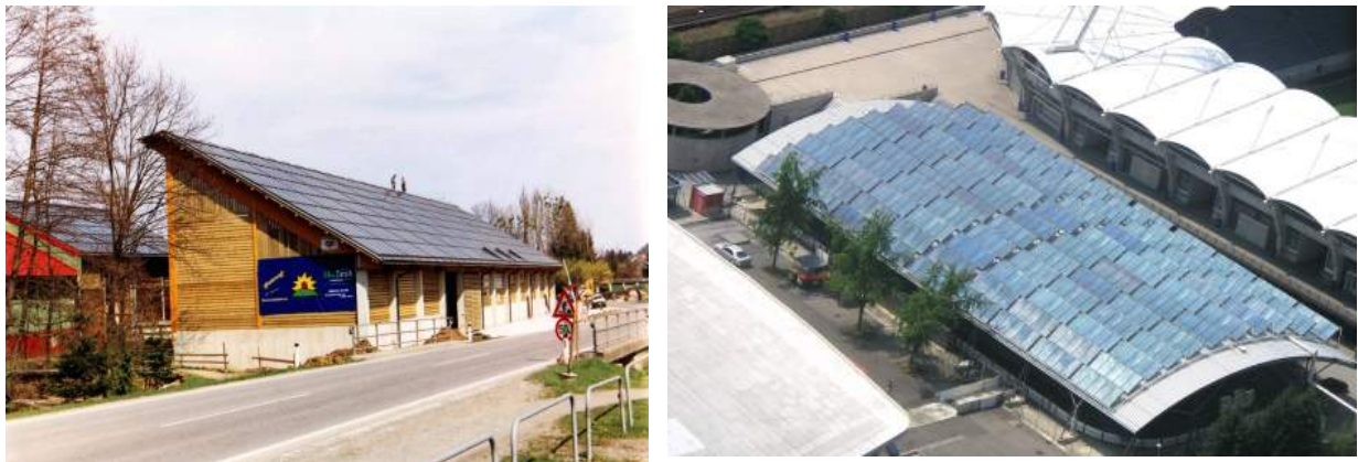
Figure 97: Left picture: Solar assisted biomass district heating plant, Eibiswald with an installed capacity of 875 kW th , (1250 m 2 collector array). Right picture: District heating plant in Graz with an installed capacity of 980 kW th , (1400 m 2 collector array). Source: S.O.L.I.D.
