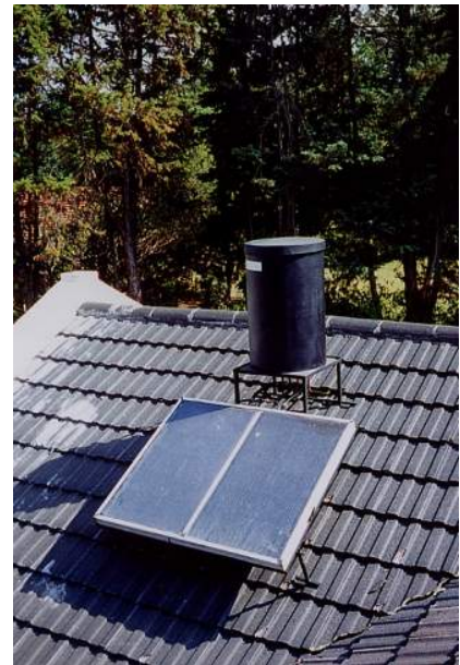
Figure 61: Non-pressurised storage tank for simple thermosyphon systems
