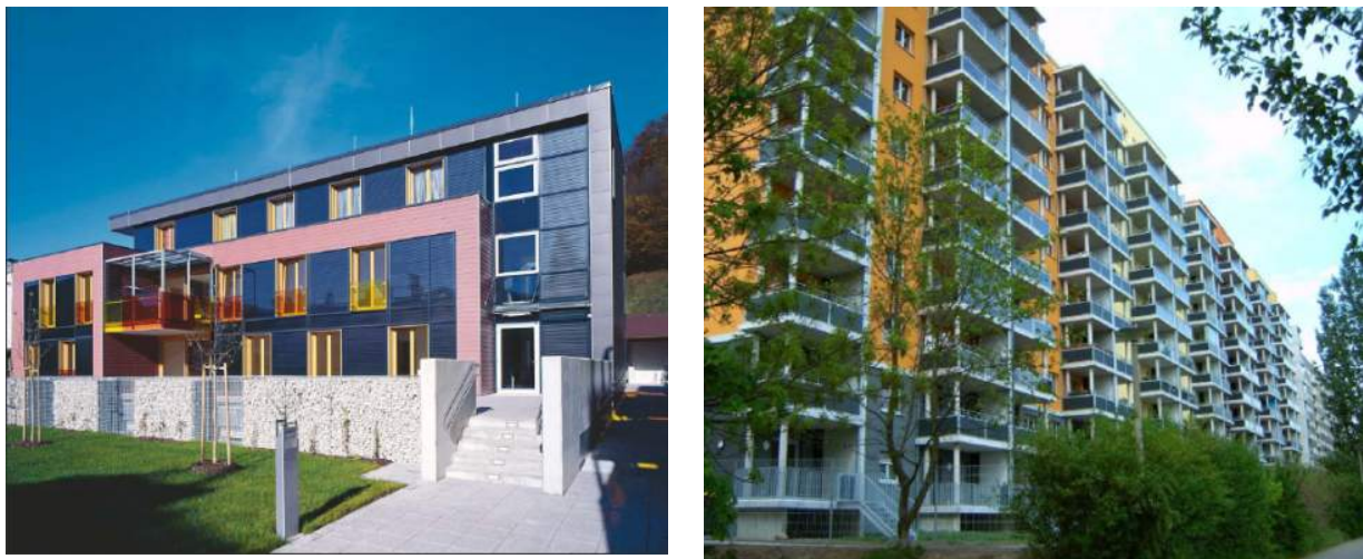
Figure 60: The façade integrated collector area has become increasingly important in the recent years (Sources: left - AKS DOMA, Austria; right: Schüco International, Germany).
