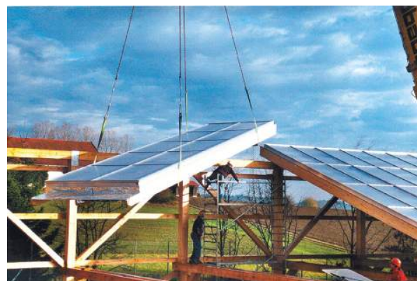
Figure 53: (left) Crane assembly of large-area collectors (picture source: S.O.L.I.D., Austria). Figure 54: (right) Crane assembly of the entire roof elements with support construction and collector field (picture source: Wagner & Co, Germany).
