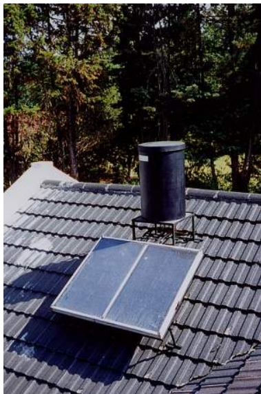
Figure 86: Simple direct thermosyphon systems, Zimbabwe
