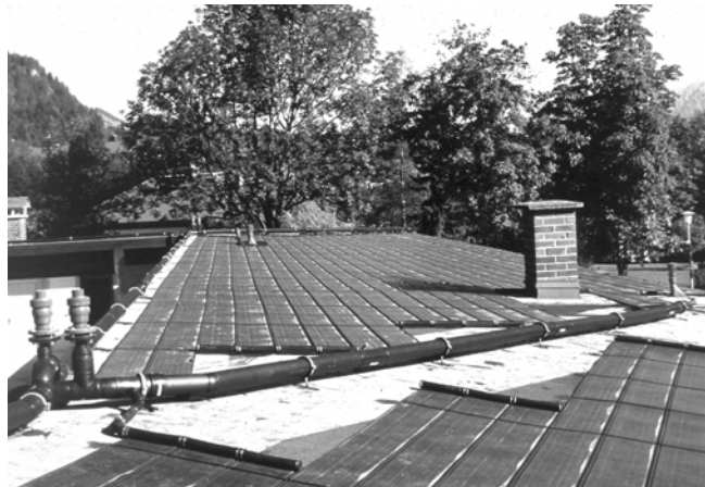
Figure 83. Solar heating system for a swimming pool (single circuit system)
