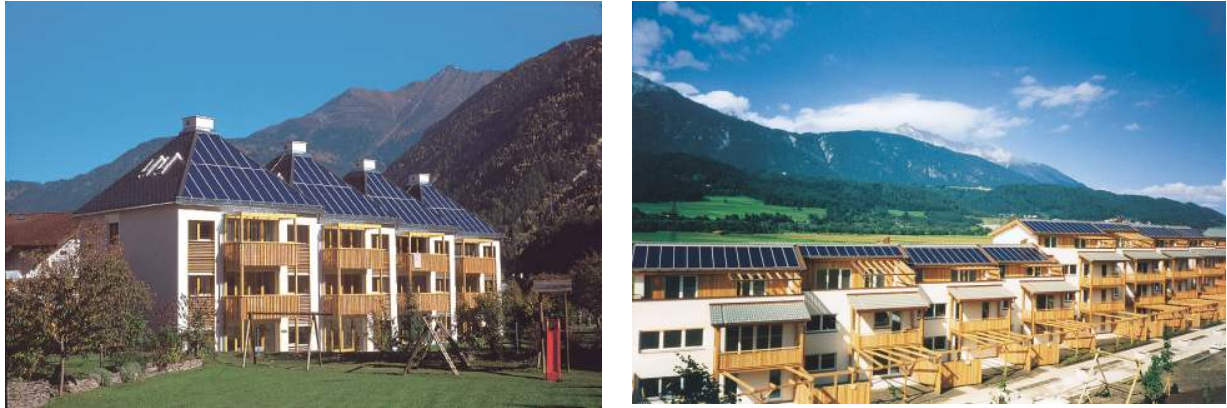
Figure 55: Roof integrated collectors (Source: Teufel & Schwarz, Austria).
