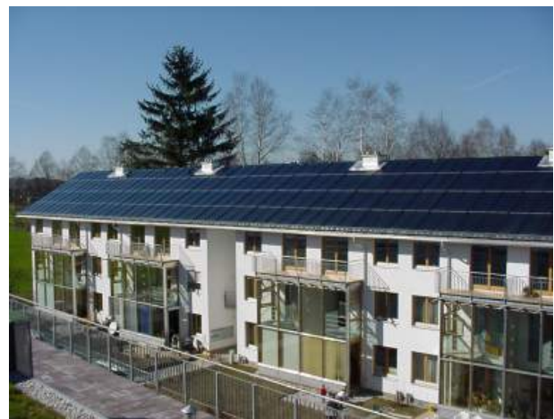
Figure 24: Flat-plate collectors on a single family house and a multi-family house
