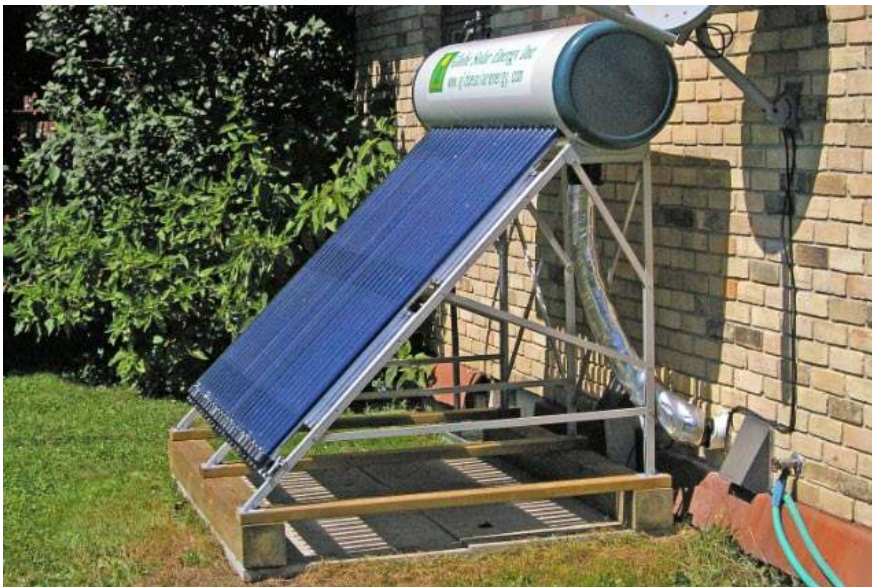
Figure 39: Thermosyphon system with evacuated tube collectors
