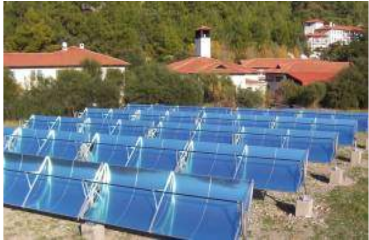
Figure 41: Parabolic trough collectors at a hotel in Turkey (Source: SOLITEM, Germany)
