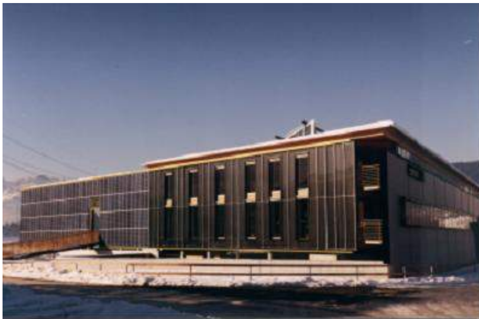
Figure 106: Solar heated production hall and office building DOMA, Austria
