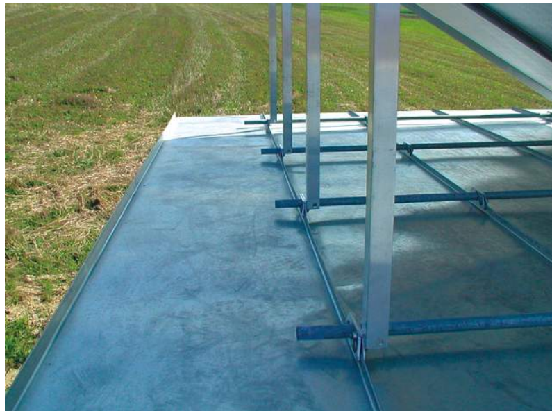
Figure 58: Clamping profiles are used to connect the collector frame to the standing seam (Source: Solution Solartechnik, Upper Austria, Austria).
