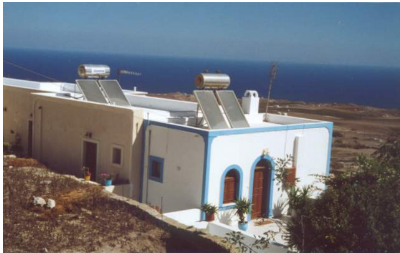
Figure 85. Gravity-driven domestic hot water system
