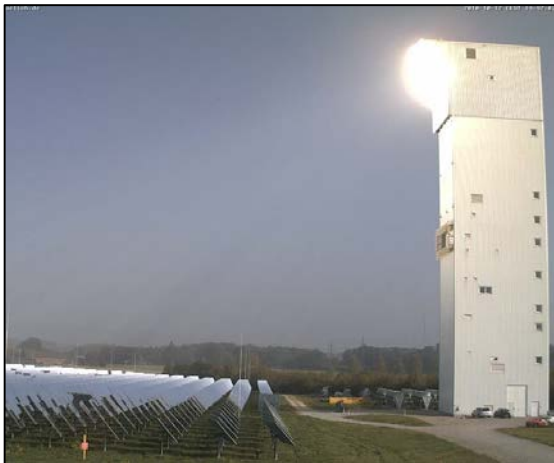
Fig 7: Solar power Tower - Jülich (Hoffschmidt, 2014)
